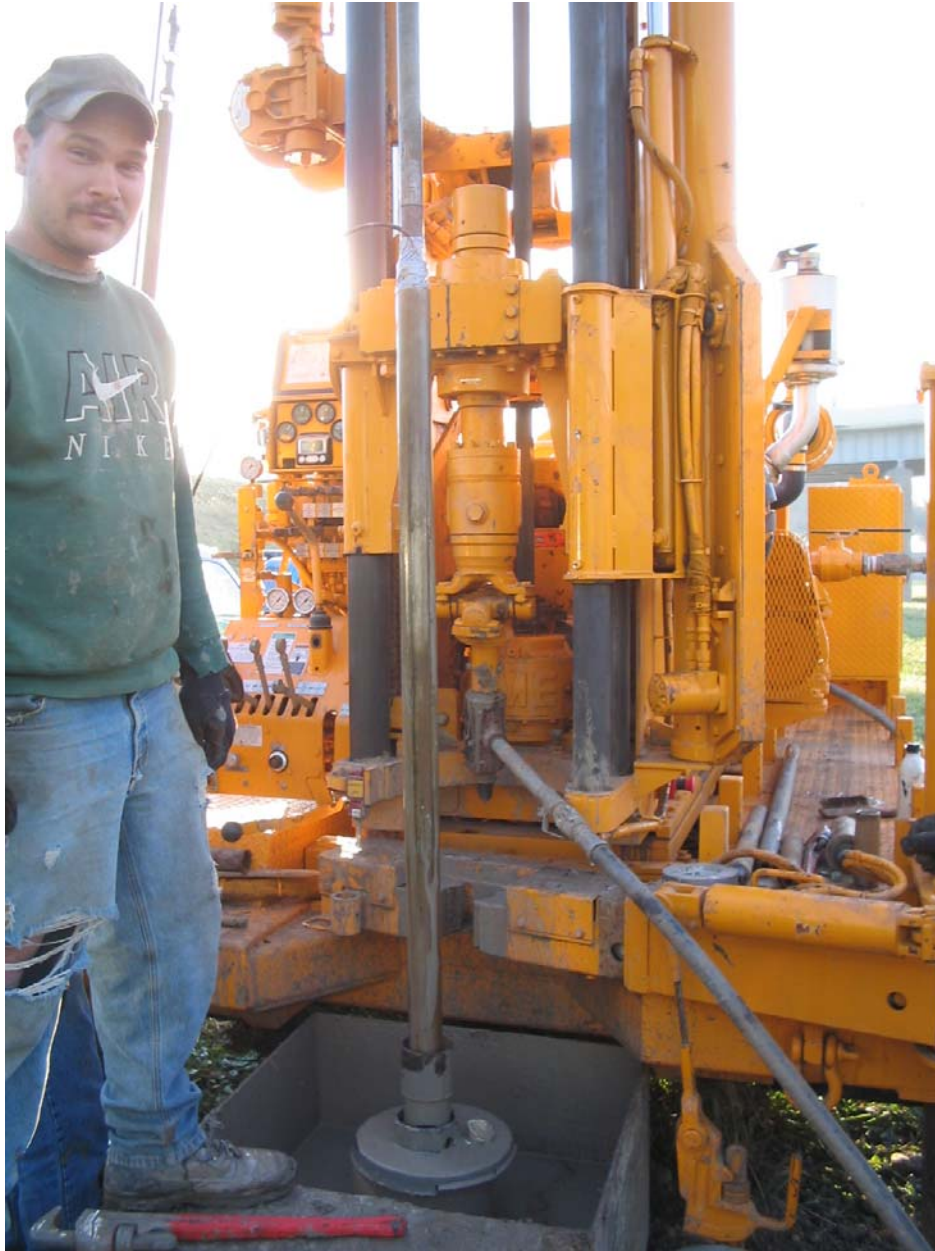
Photo 1. Lowering the slotted casing PMT into borehole (Lee, 2004)
