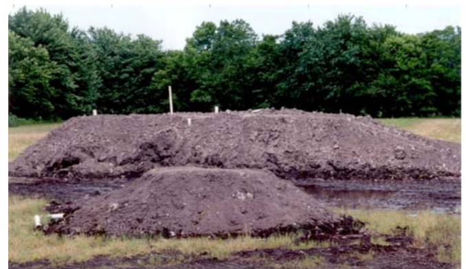
Figure 6: Embankment load test setup
